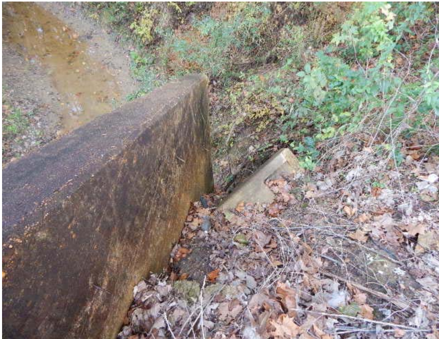
ABUTMENT 1 RIGHT WING WALL (WASHING BEHIND)
