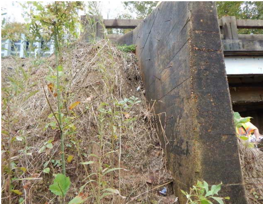
ABUTMENT 2 LEFT WING WALL (WASHING BEHIND)
