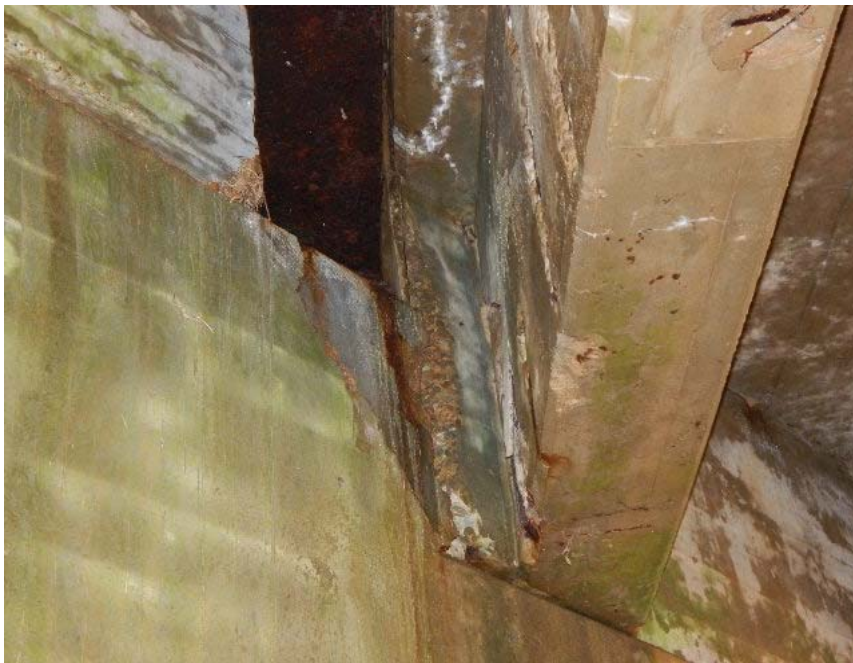
BREAST WALL- IMPENDING SPALL UNDER BEAM "H"
